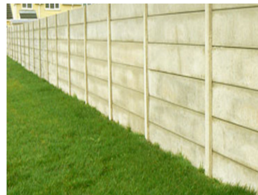
Concrete Post & Panel Fence
