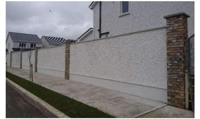
Block Wall with dashed finish and brick piers 2m high - Durkan Site
