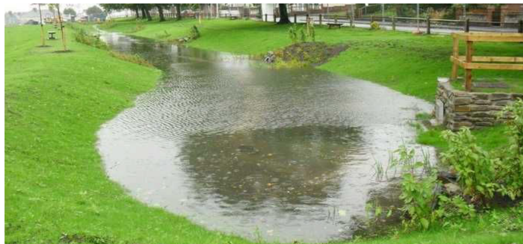
Typical swale in wet weather
