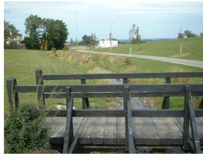
Pedestrian Foot Bridge
