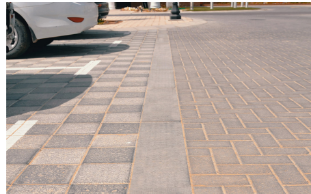
Flush Slipform Concrete Kerb
