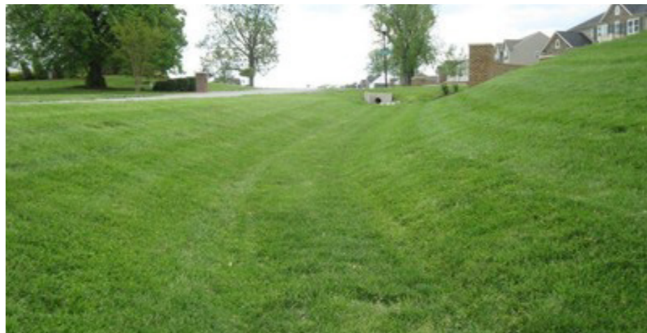
Typical swale in dry weather
