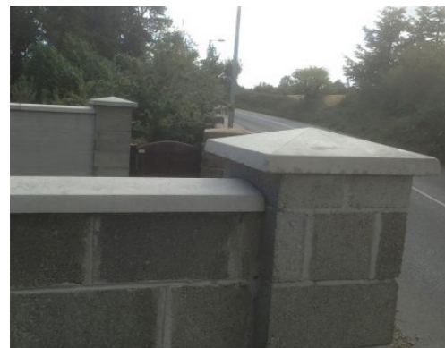
Fair-faced Concrete Wall
