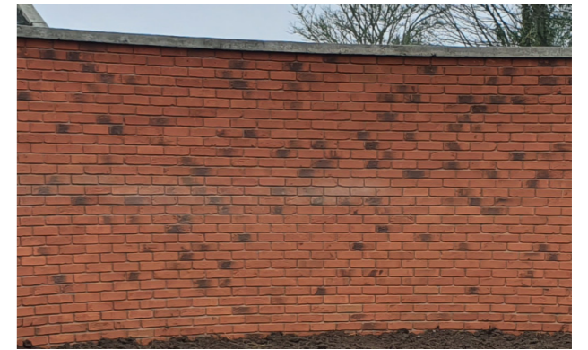
Brick Feature Wall 2m high - Kelland Site
